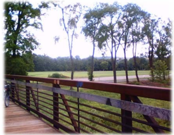
Figure 5: Pedestrian Bridge between Glendale Park and River Bend Park
